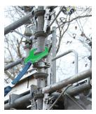
Proper tie off to vertical leg up to 6ft above wrapped bay using hook **side-rated at 3,600 lbs.**
