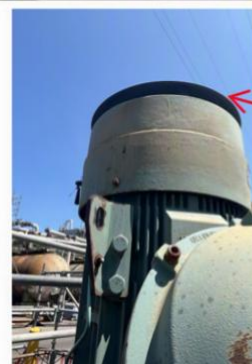
Sharp edge of motor that caused rigging damage
