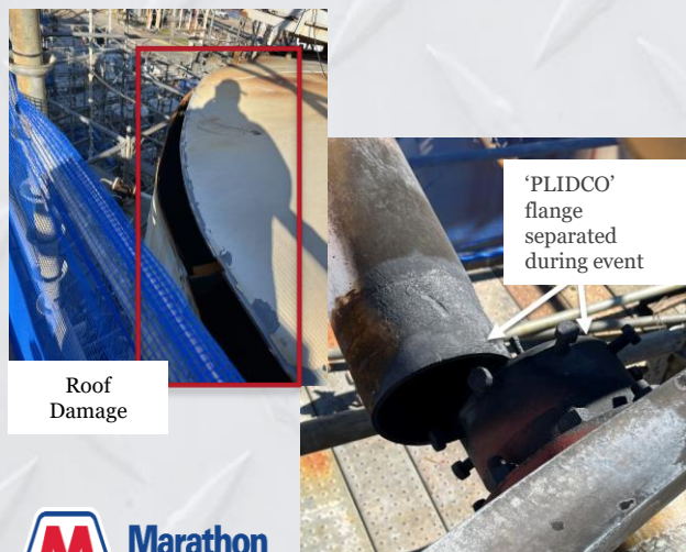
INC 409438: Sour Water Facility Tank 222
