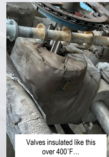
Insulated flange location
